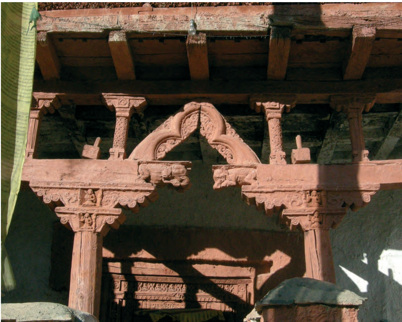
Fig. 15: Central part of the veranda construction with a triangular centrepiece and elephant consoles, the top lintel of the door in the background; photo CL09 D5340.
