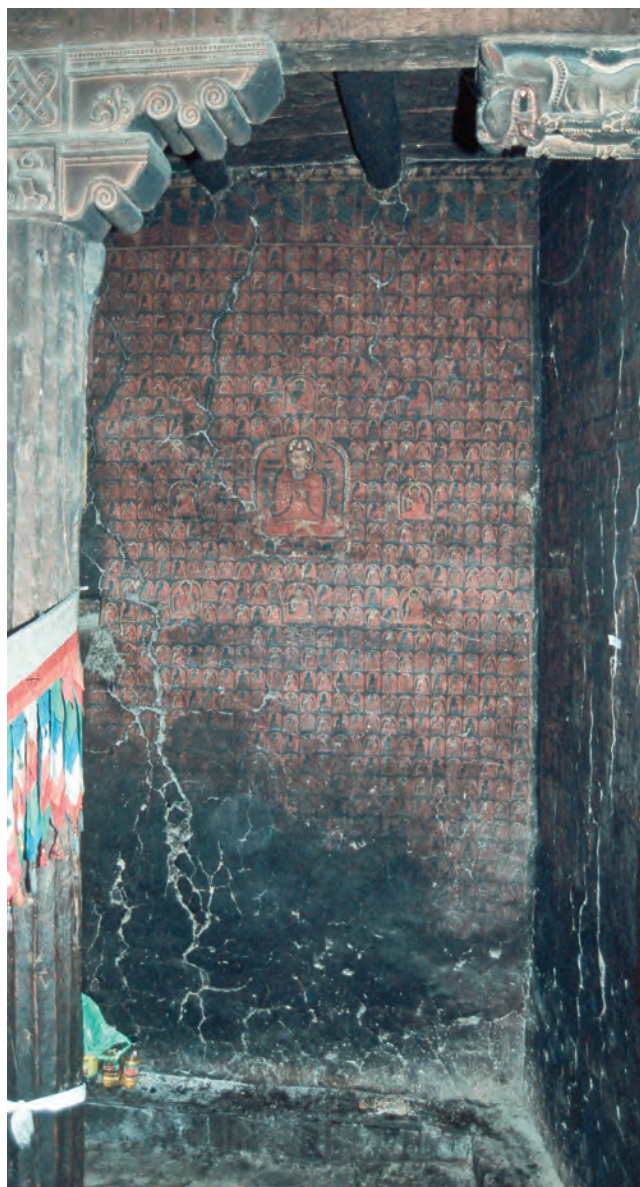
Fig. 194: General view of the wall to the right side of the entrance.
