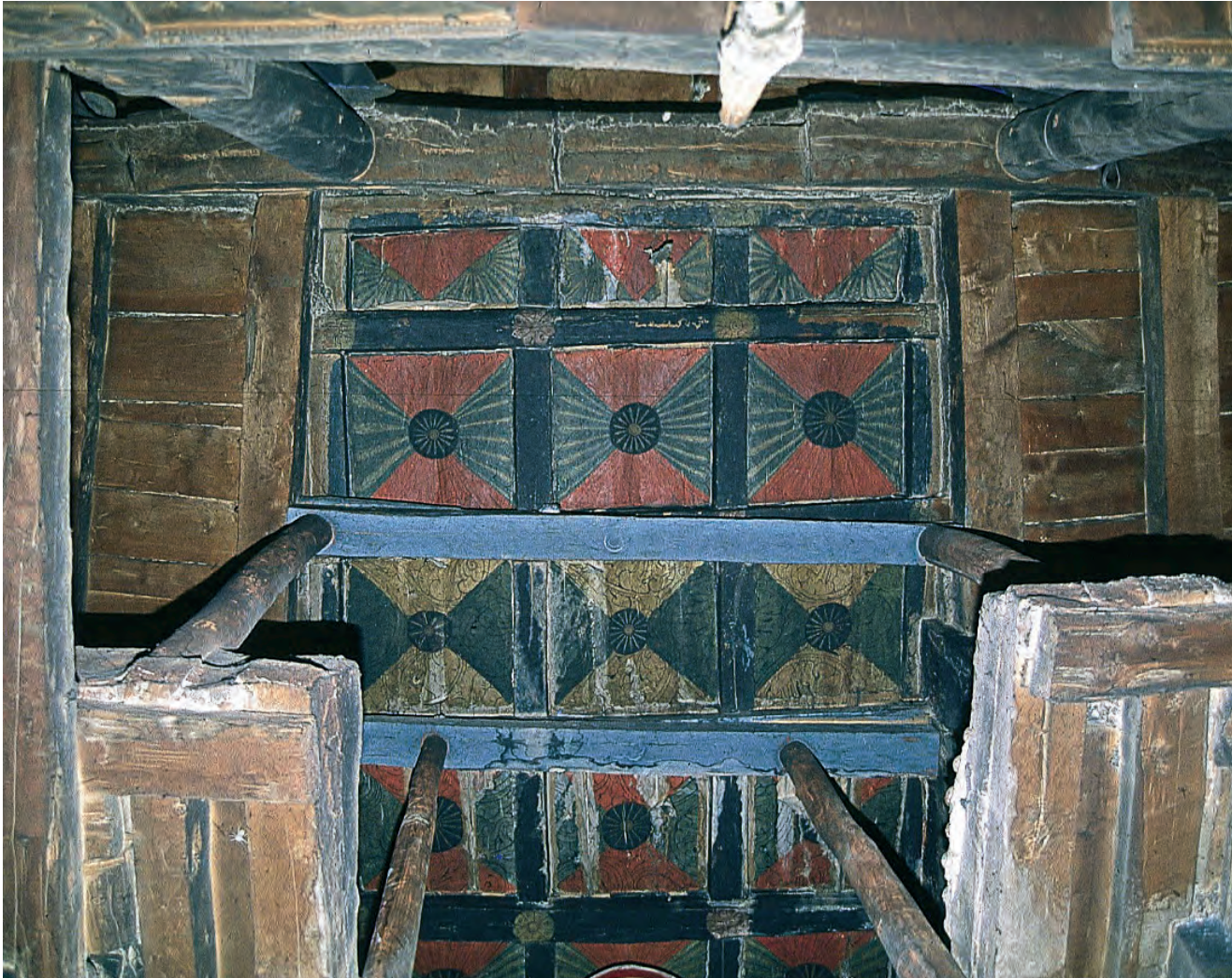
Fig. 37: Only the ceiling of the main niche and the area immediately in front of it is decorated. This area is constructed as false cassettes with painted textiles pasted into it's squares.
