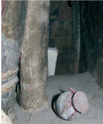
Fig. 44: At the back of the large sculptures some details of their construction are visible. The images are built around a massive vertical post. On the pedestal lies the flask attribute Maitreya originally held in his hand.
